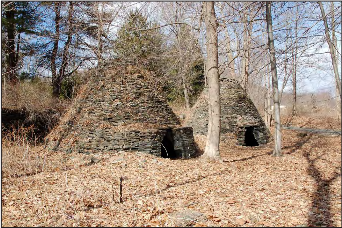
PHOTOGRAPH 19: Wassaic Charcoal Kilns, View to Northwest
